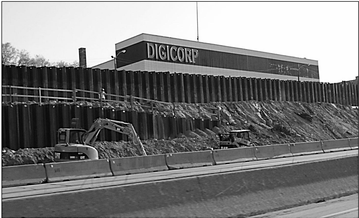
Sheet pile wall
