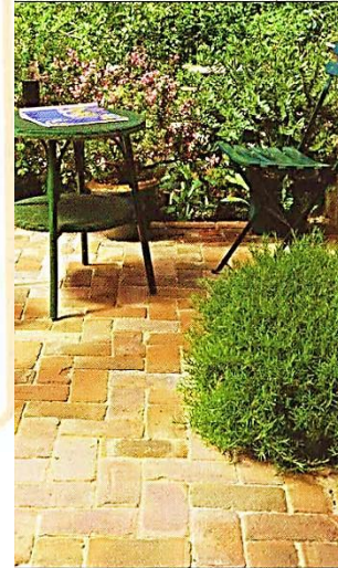
A traditional patio made from high-fired bricks. The herringbone design – with the bricks set square to the sides – keeps brick-cutting to a minimum.
