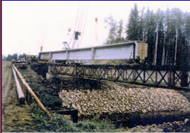
7-9 Using a launching truss for girder erection
