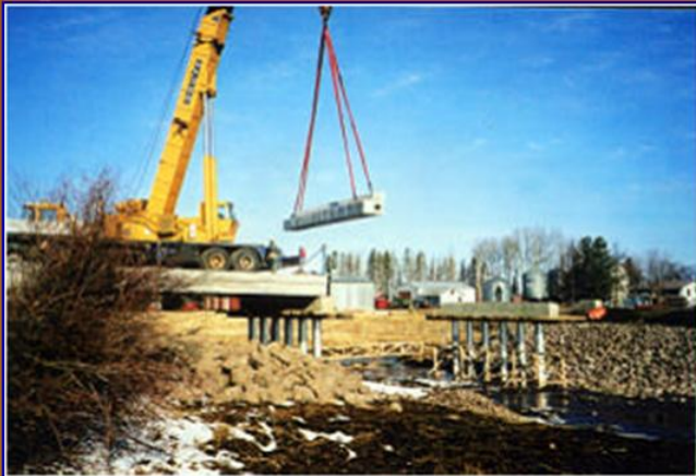
7-11 Erecting middle span girders on top of previously erected first span girders
