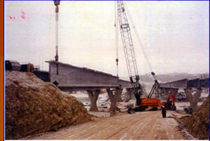
7-2 Hoisting precast concrete girder into position with two crawler cranes
