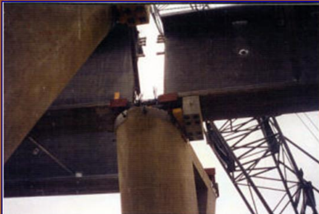
7-3 Girder on temporary bearing at pier
