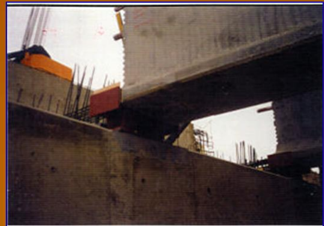
7-4 Girder on temporary bearing at abutment
