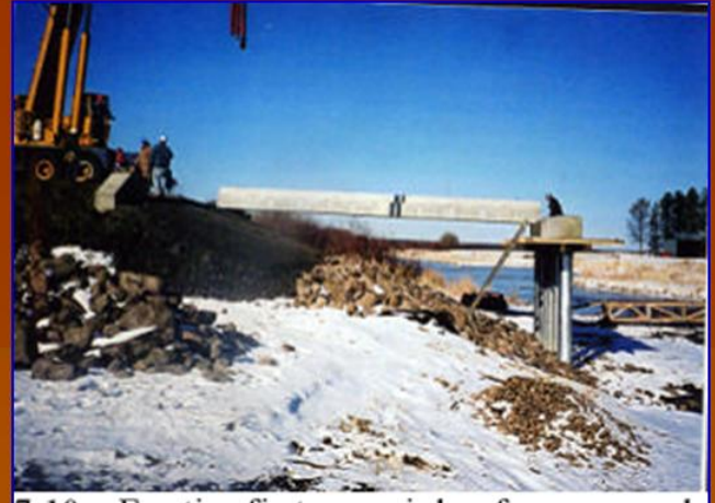
7-10 Erecting first span girders from approach
