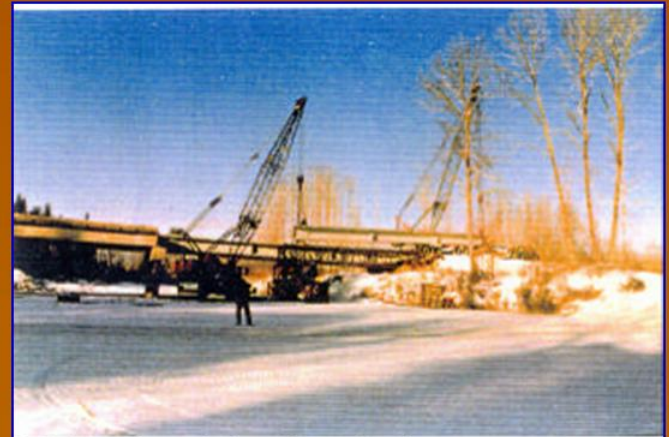
7-8. Erecting girders from the ice
