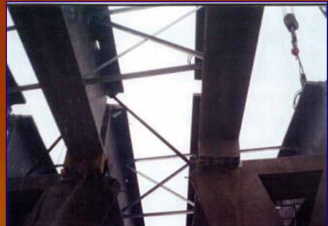
7-6 Subsequent girders erected, stabilized with permanent steel diaphragms
