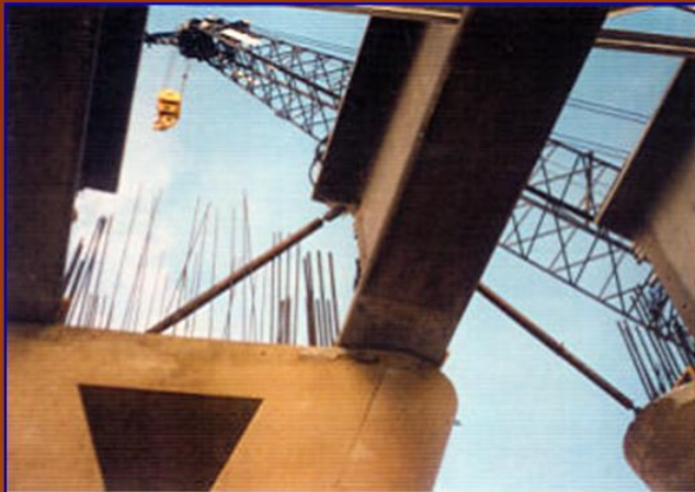
7-5 First girder erected, stabilized with temporary shoring
