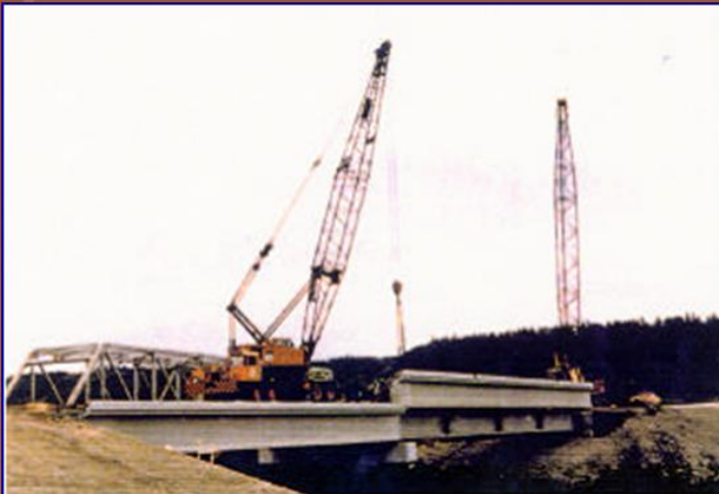
7-7 Erecting girders on top of previously erected girders
